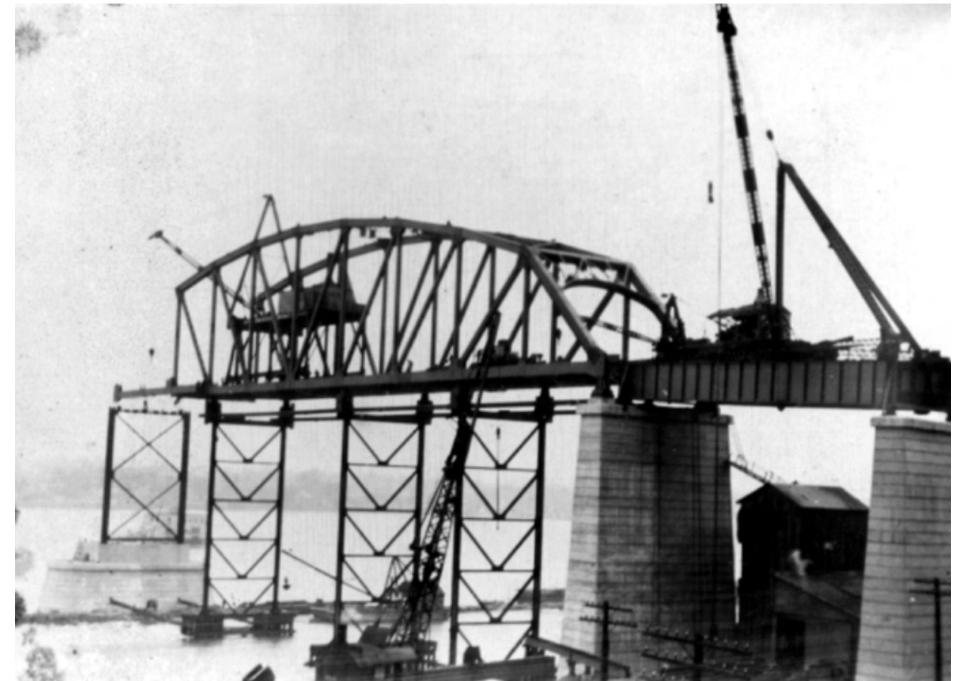
Peace Bridge under construction.
