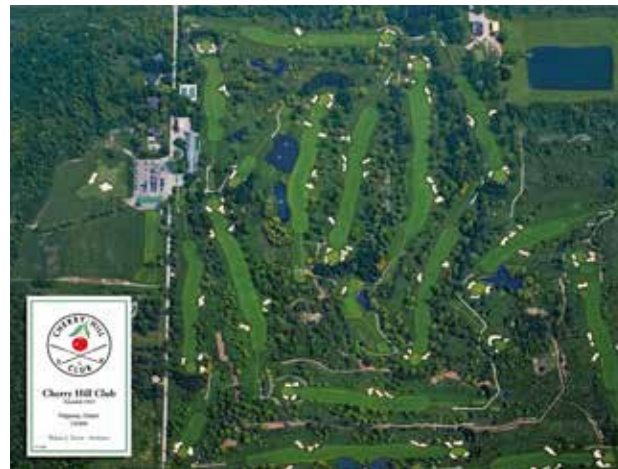
Pre-renovation aerial shows plethora of bunkers. Drainage ditches are also visible.
