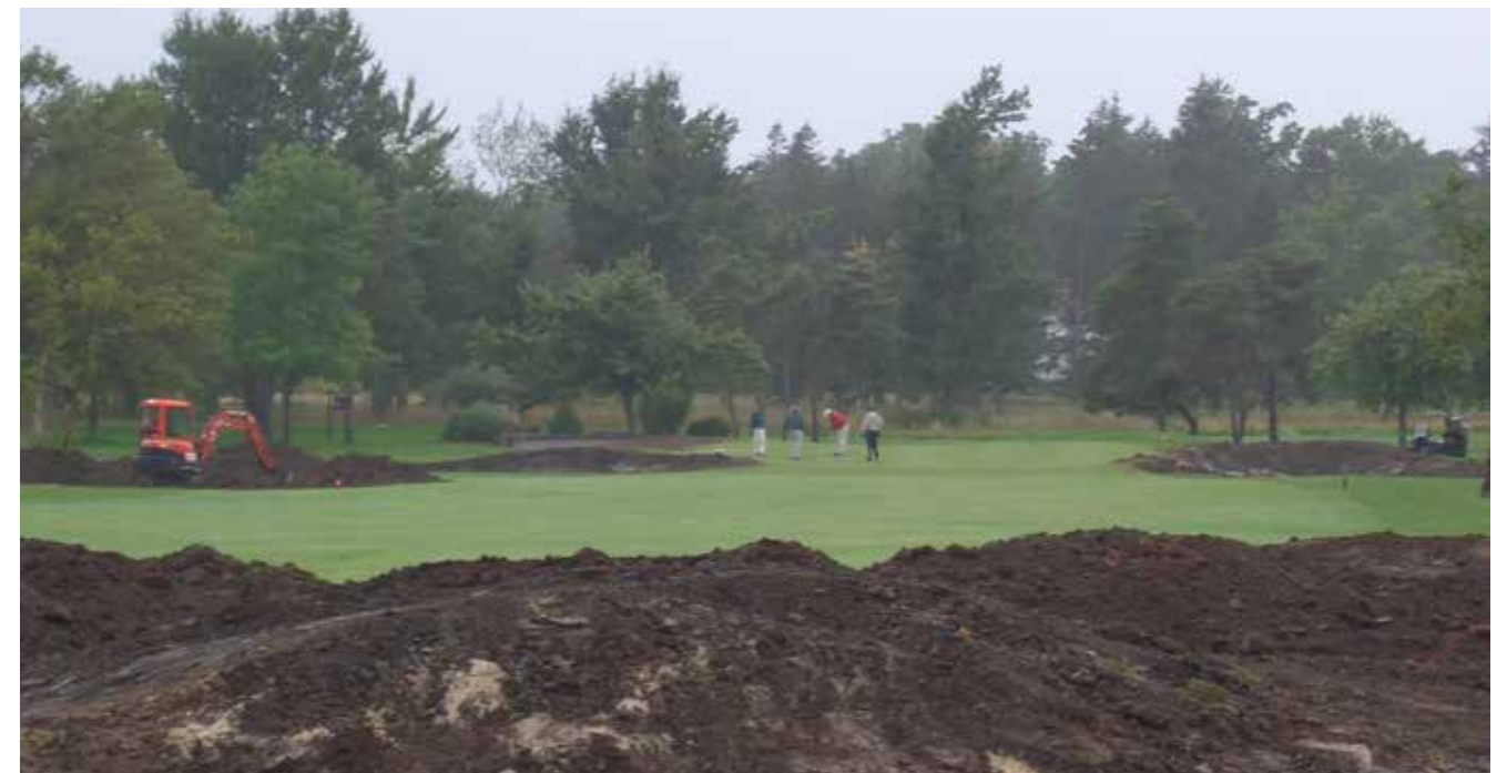
The course remained mostly open for play during the renovation.
