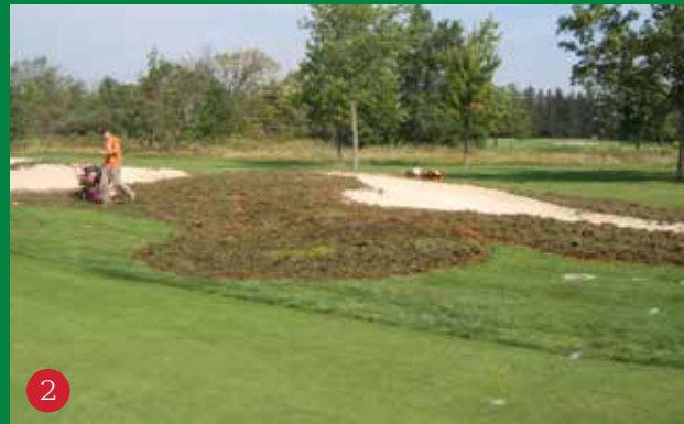
2 Ground is prepared for the new bunkers.
