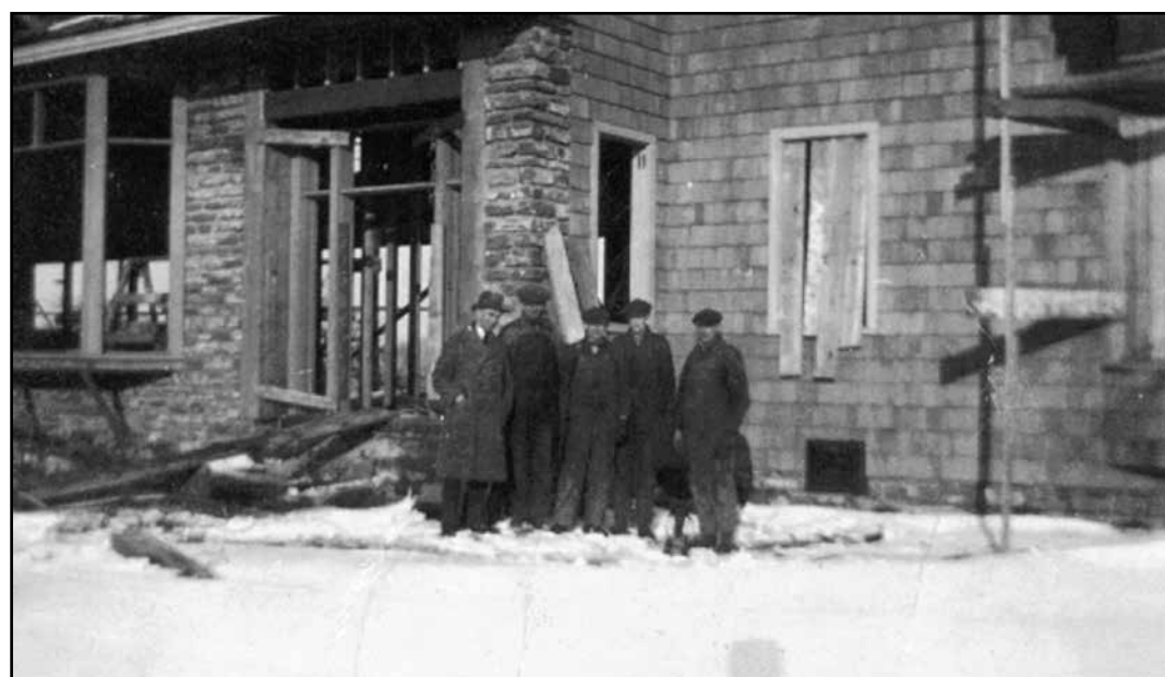
Albert D. Nie and crew, of Fort Erie, contractor for the Cherry Hill Club c. 1923.
