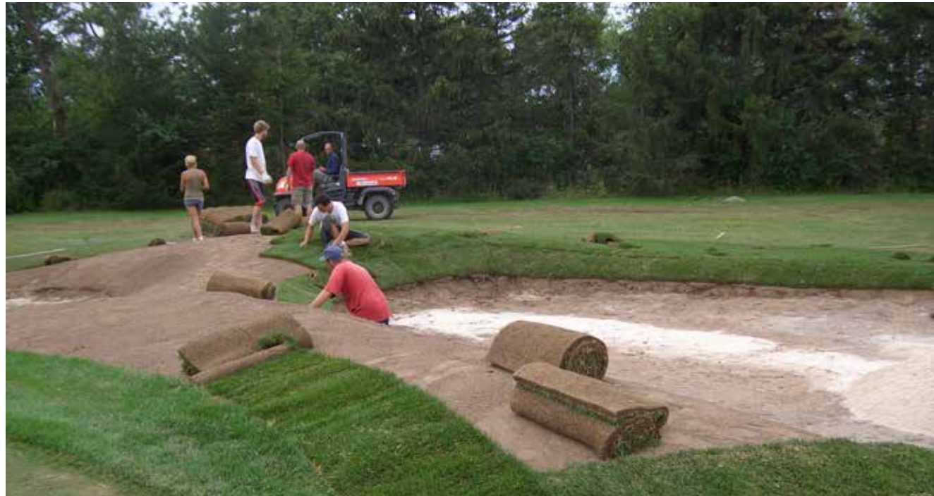
The NMP Golf Construction crew sods a bunker on hole #13.
