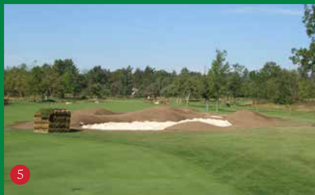
5 New sand is placed, and mounds are ready for sodding.
