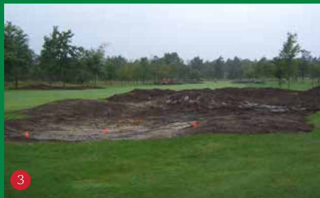
3 After sand removal, fill is piled in rough configuration.
